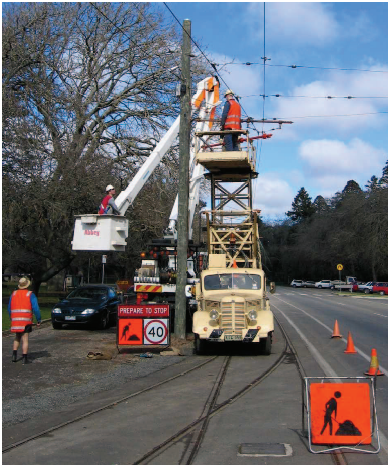
Pole and bracket arm replacement with the assistance of Powercor. 16 August 2005.
